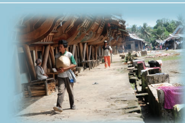
Omo Hada The understructure or the supporting columns are the strength points of Omo Hada , the traditional dwelling-house of Niassan. The wooden vertical supporting columns ( ehomo ) and the diagonal supporting columns ( ndriwa ) of Omo Hada (traditional Niassan dwelling) rest upon stone boulders. This allows flexibility for the house to move or shift following the quake's horizontal force in the event of an earthquake.
