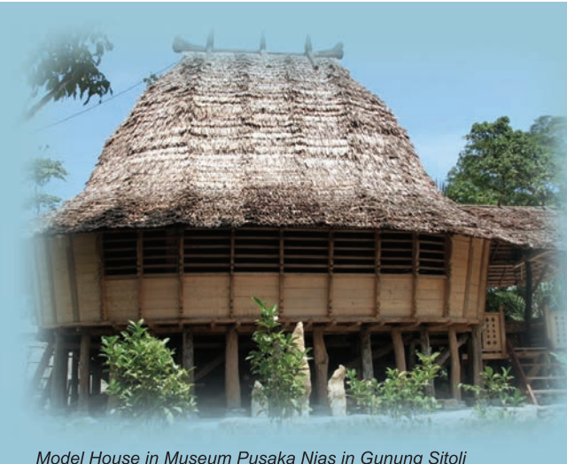
North Nias Traditional House Traditional houses in North Nias District are oval in shape. We can see fine examples of North Nias traditional houses in Tumori Village near Gunung Sitoli. These houses have more complex earthquake shock resistance structure system.
